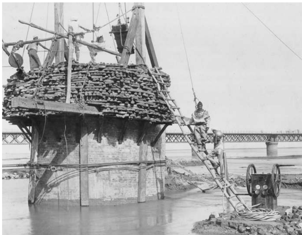
BB_023 - a diver and his breathing apparatus beside one of the weighted piers.
